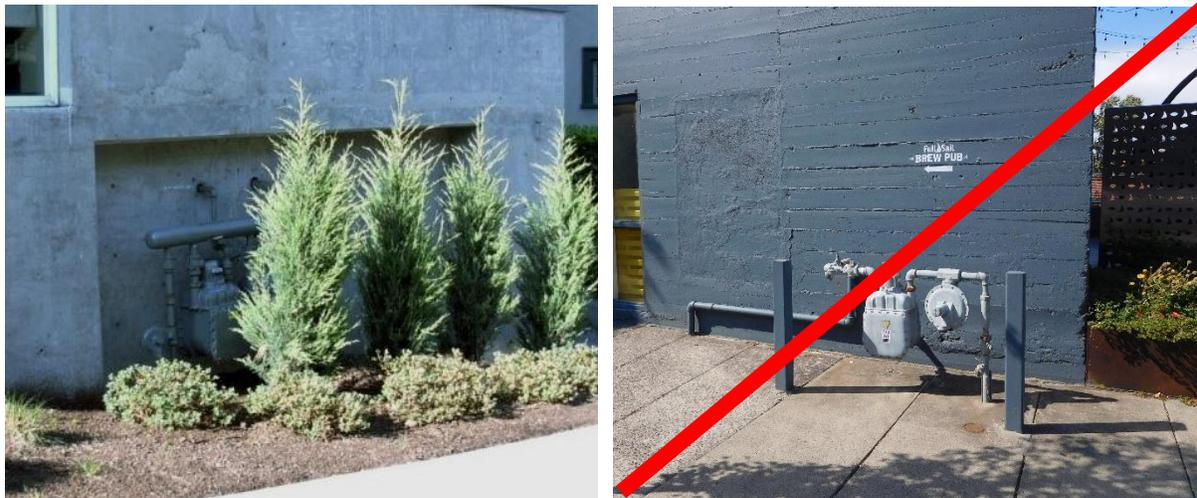
Place utility meters in less visible locations. The left examples is successfully tucked away in a less visible location and screened by vegetation. The right image is poorly executed and would not be permitted in such a visible location; such meters must be coordinated and better integrated with the architecture of the building.
