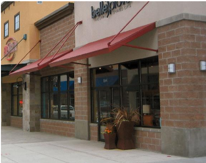
Figure 3.4.A Acceptable concrete block use/design.
