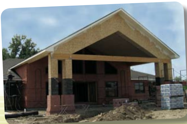
The first of three new medical office buildings.
