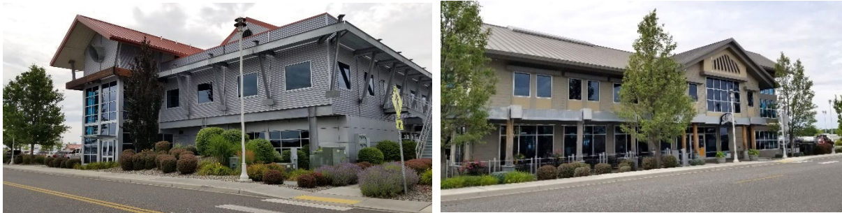
Examples of existing Port buildings.
