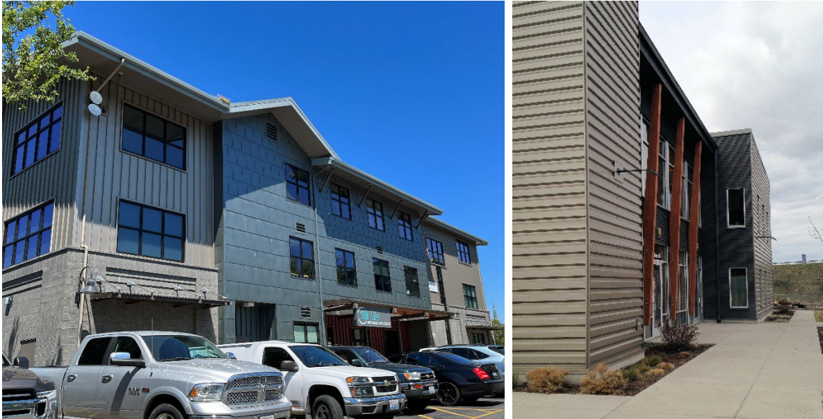
Figure 3.5.C Acceptable metal siding examples.
